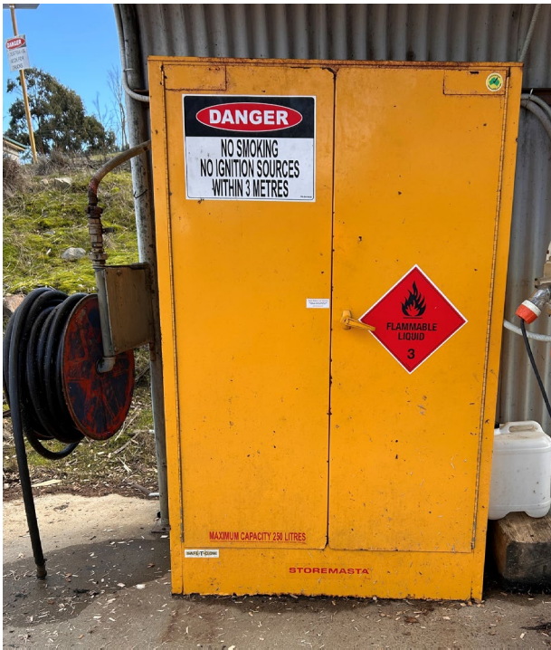
Figure 18 Flammable substances storage at Longreach Mill
