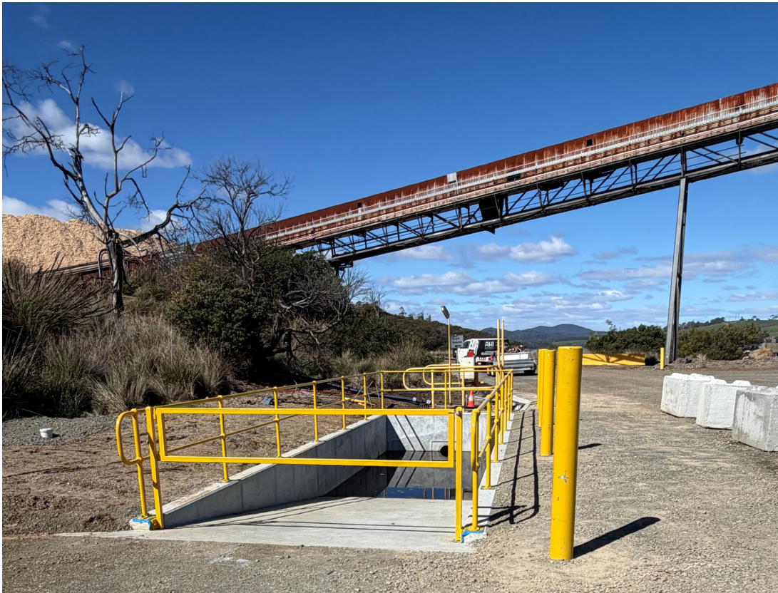
Figure 19 Upgraded drainage pit and leachate located adjacent to the wharf.
